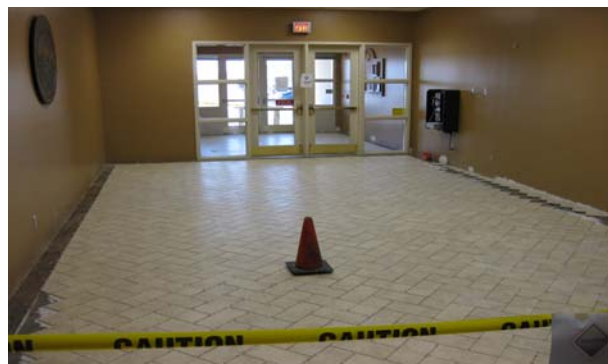
Figure 1 – Tile Project in Administration Building
